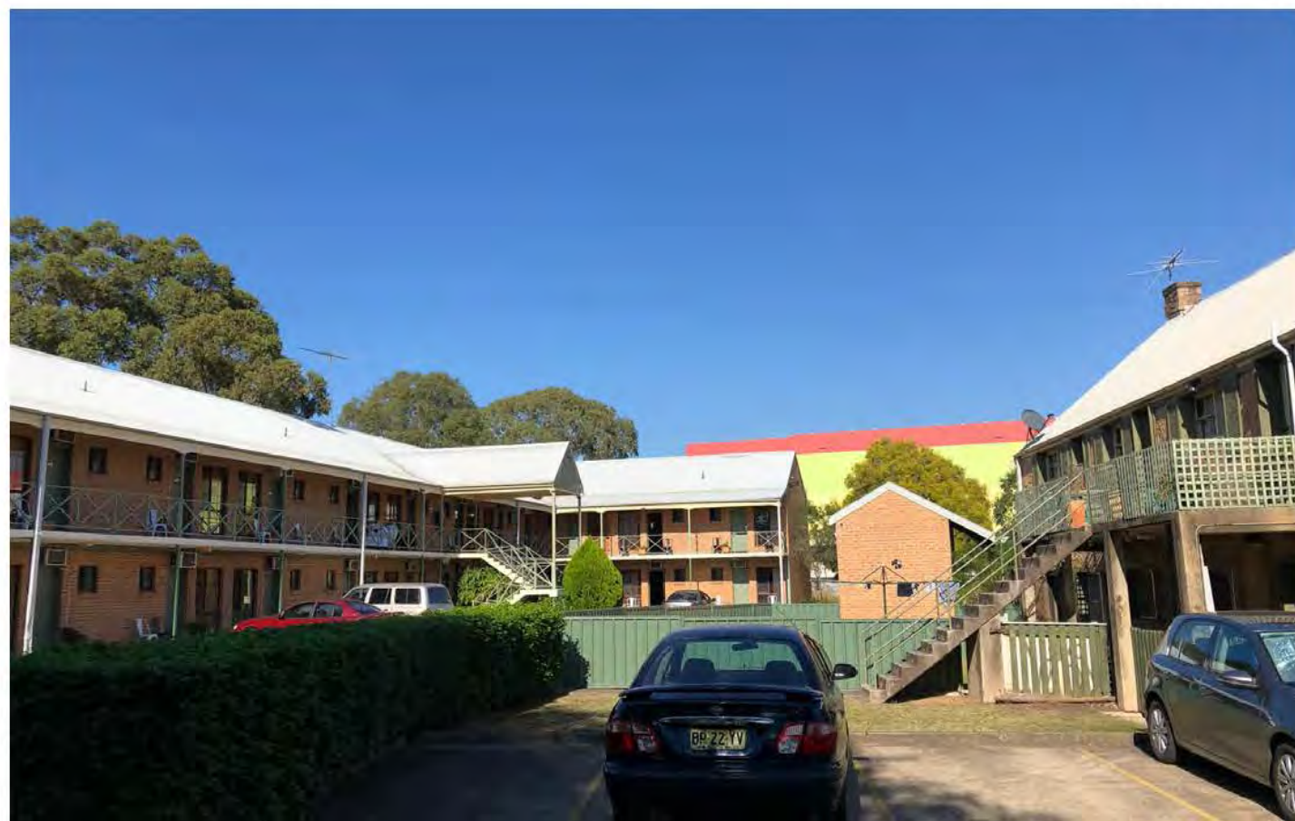
Interface with recent motel development
