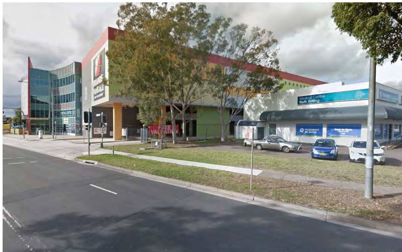
View from Queen Street - Subject Site
